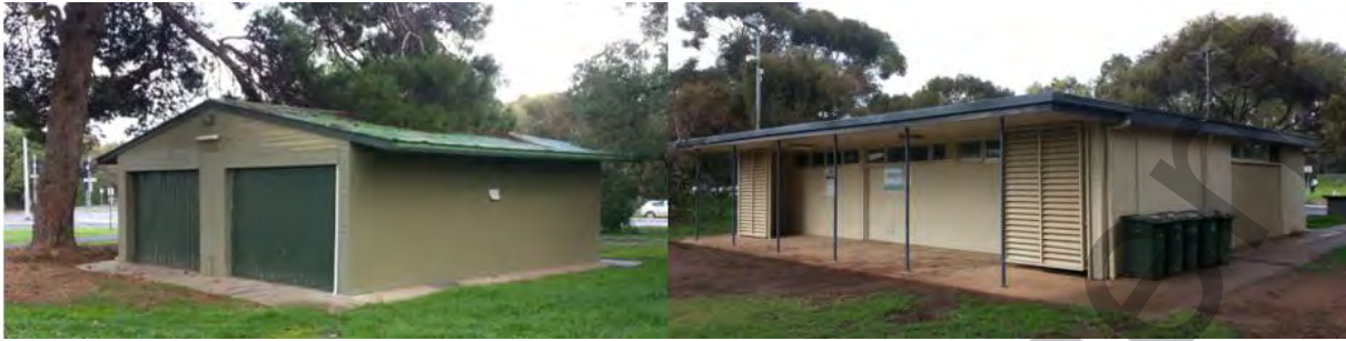
Existing Buildings in Park 9
