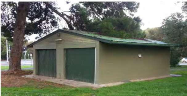
Existing Maintenance Shed
